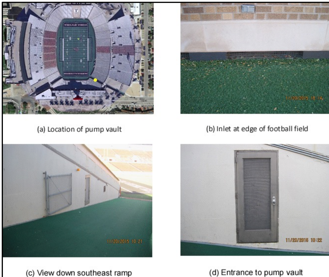
Figure 1. Photographs of Lift Station Location and Field Inlets
