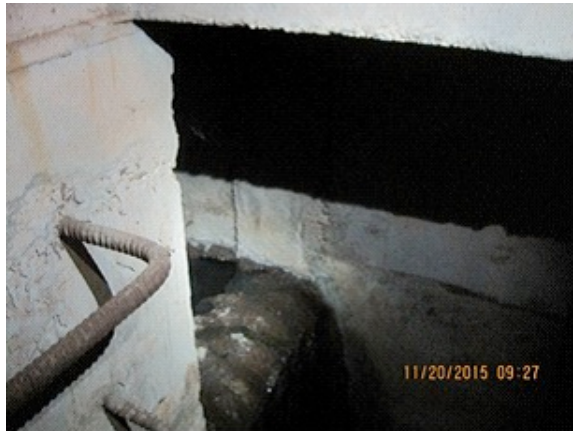
(a) Overflow weir into sump
