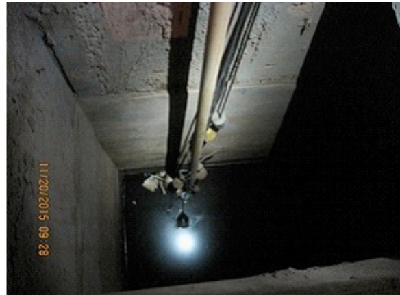
(b) Looking down at float actuators
